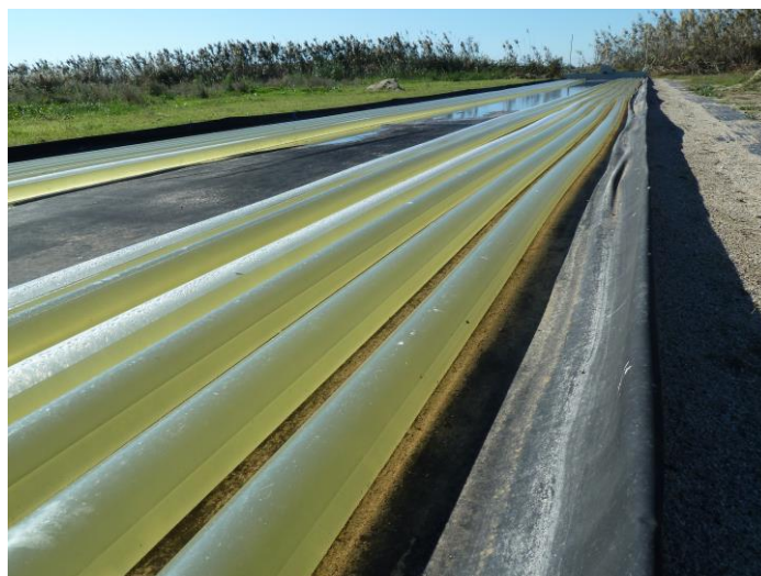
Photo 2. Image of horizontal pipes that make up the return circuit
