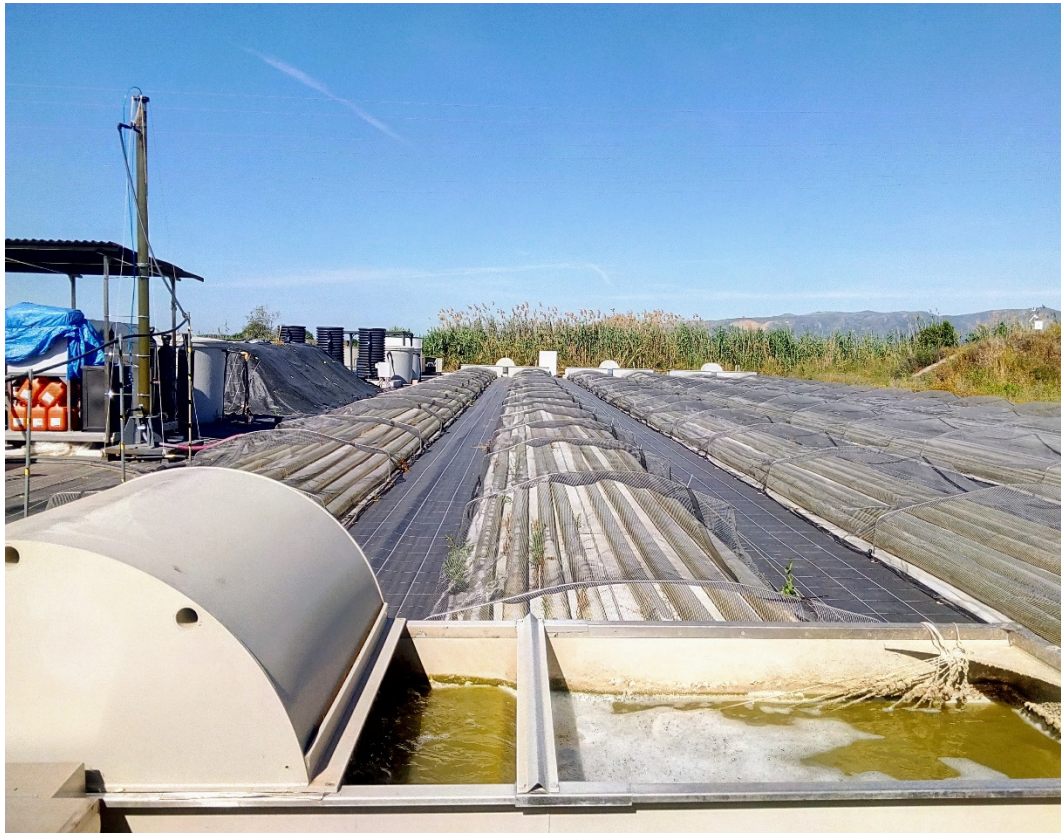
Figure 15. View of the biogas upgrading column, located between the anaerobic (co-)digestion plant and the third photobioreactor.
