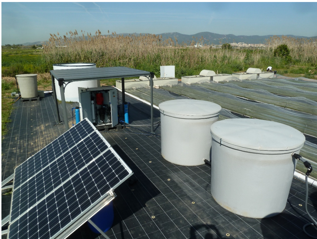
Figure 17. Solar-driven filtration and disinfection unit: feeding tanks (right), compact box containing the filtration, disinfection and control devices (under the roof), and photovoltaic solar panels (left).
