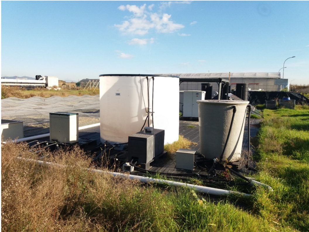
Figure 6. Tank for mixing and homogenization of the influent wastewater.
