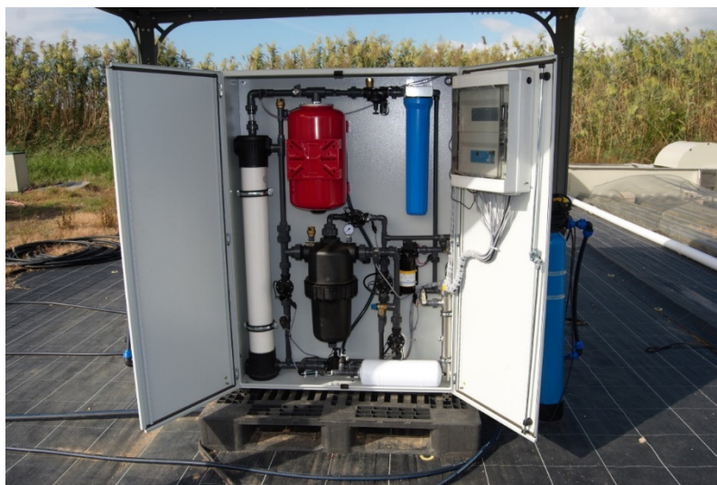
Figure 18. Detail of elements and devices for filtration and disinfection contained inside the box.
