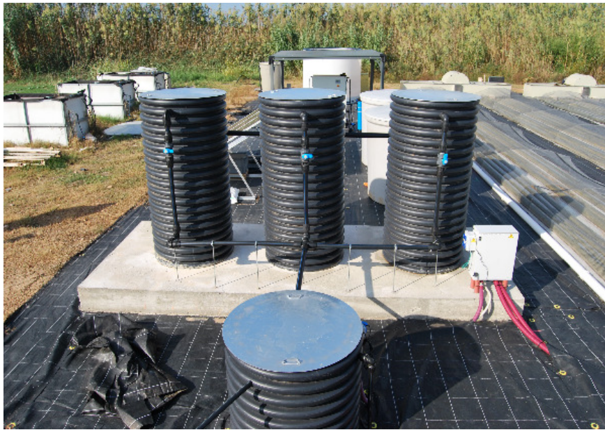
Figure 19. Adsorption columns for phosphorus recovery.
