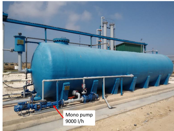
Figure 1.12: Anaerobic co-digestion system.
