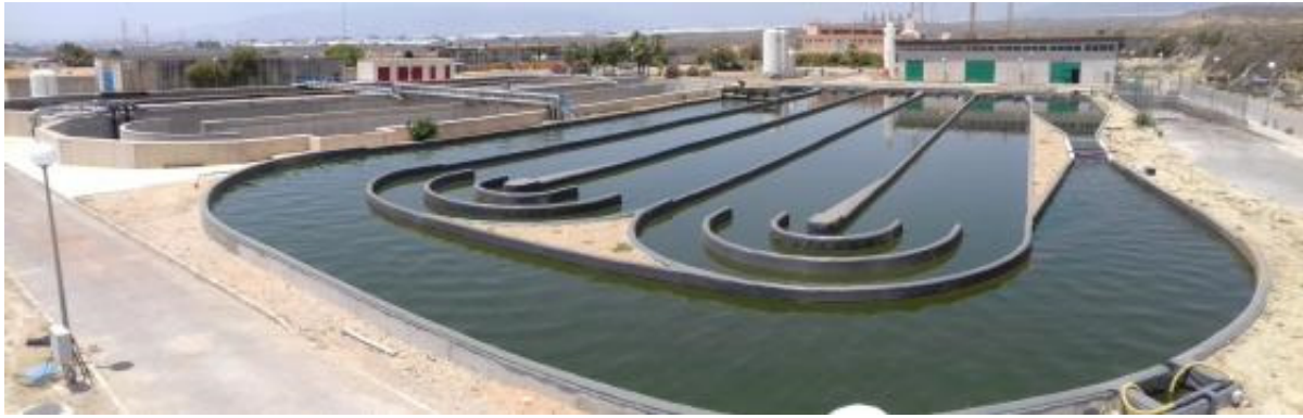
Figure 1.16: High rate algae pond of 3000 m2 under construction (above) and full operation (below)
