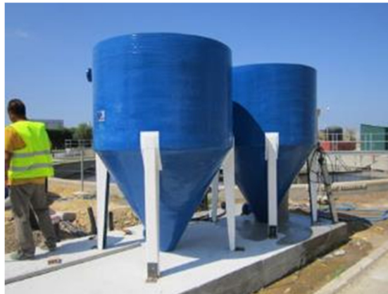
Figure 1.7: Clarifiers for PPBs separation.
