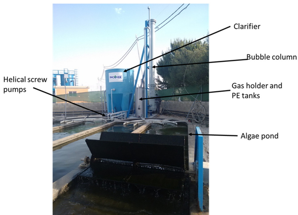
Figure 1.13: Photosynthetic biogas upgrading at El Torno WWTP.
