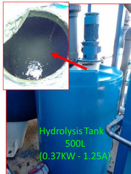
Figure 1.11: Hydrolysis tank for anaerobic pretreatment.
