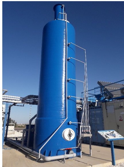
Figure 1.3: New PUSH reactor.
