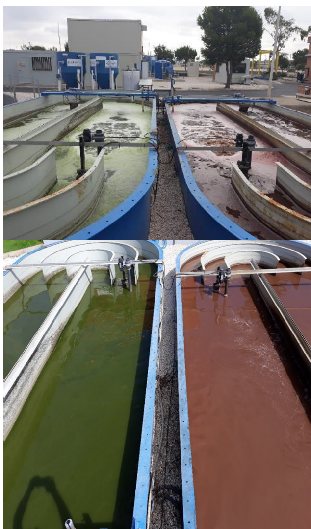
Figure 1.6: POND 1 and POND2 DEMO for VFAs production at Chiclana with and without aeration. Purple bacteria in pond 1 (right).
